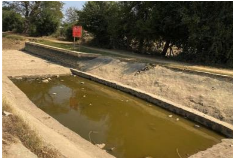
Figure 8. Irrigation canal in Sint Kai Township with lower level of water
